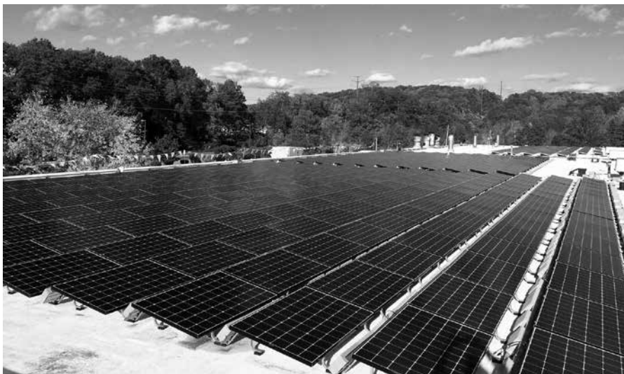
The roof mount is on top of UPS building in Waterford.
